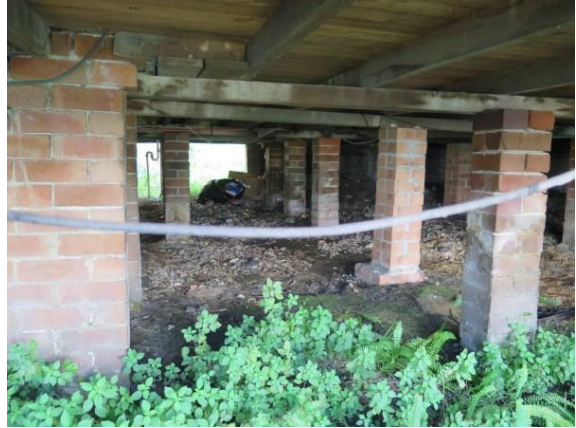
Figure 3.18 Brick footings beneath 2 Thomas Street. (Source: GML, 2016)
